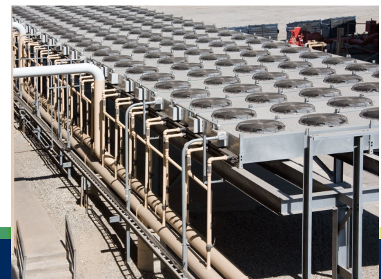
Air Cooling Fan-Array. Source: EvapCo
